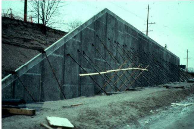
Highbury Avenue propped panel wall, London Ontario, 1989 (Bathurst 1993)
