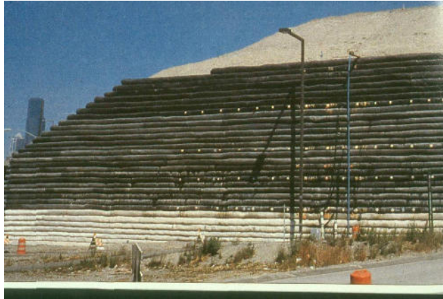
Rainier Avenue Wrapped-Face Geotextile Wall (Seattle, Washington, 1989)
